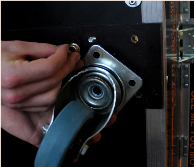
On the outside, slide the screws into the wheel.
